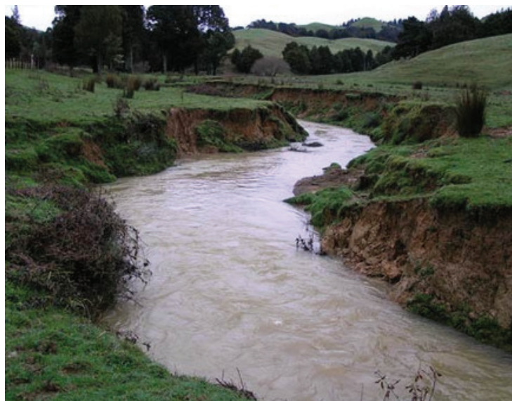
Figure 1. Stream bank erosion.
