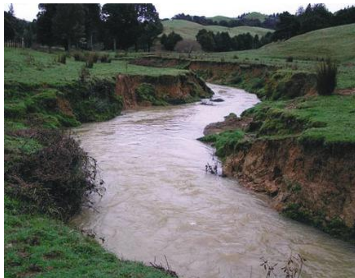
Figure 1. Stream bank erosion.
